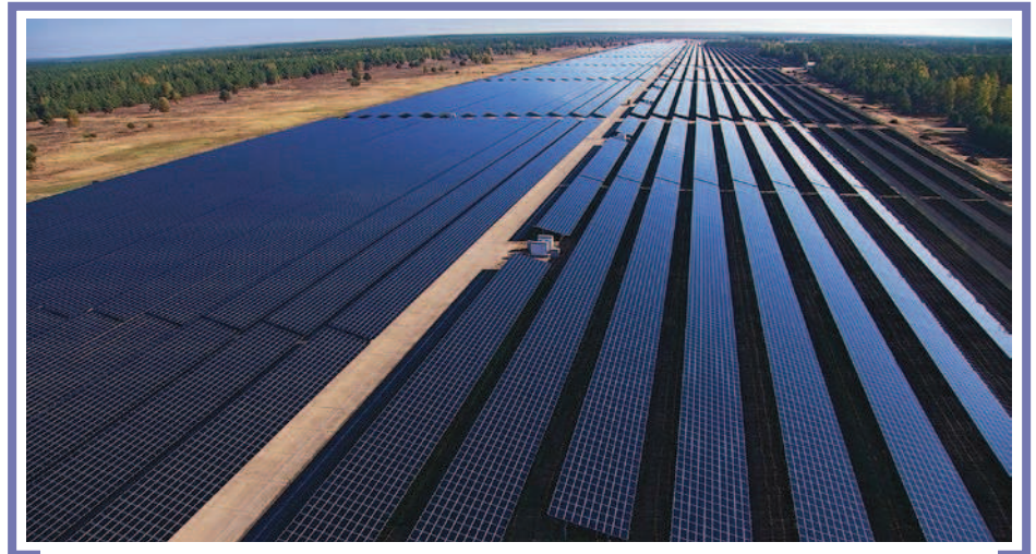
Thin-layer in rows: solar project developer Belectric has built Europe's biggest photovoltaics power plant in Eastern Europe using cadmium-telluride modules by First Solar.
